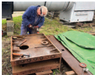
A volunteer takes the wire brush to the drag box. It will be rivetted into place between the loco's frames beneath the cab.
