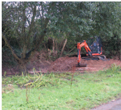
Excavating the pond at the Knapp
