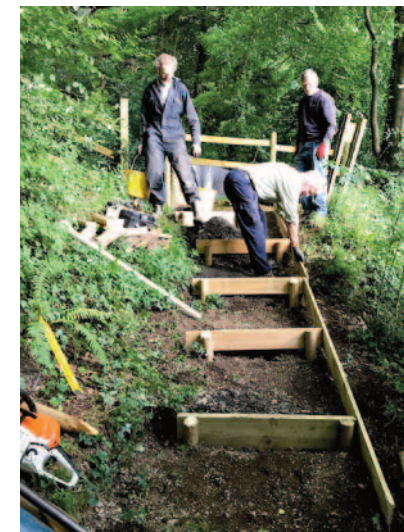
New steps on Footpath 116a leading off Salcombe Hill Road.
