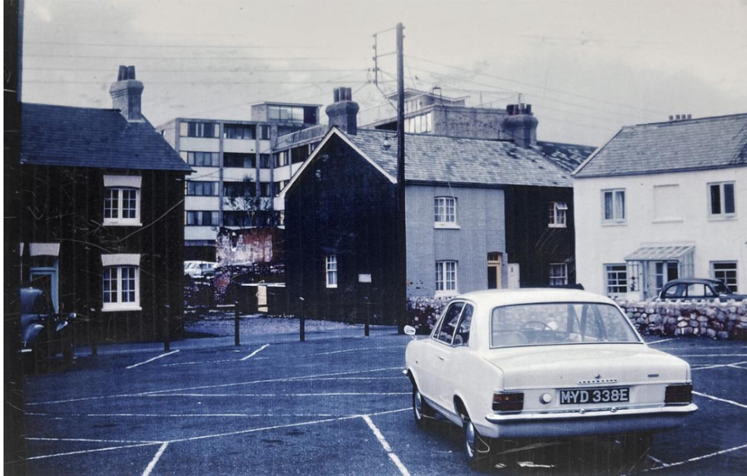
View from Ham East car park, behind the swimming pool
